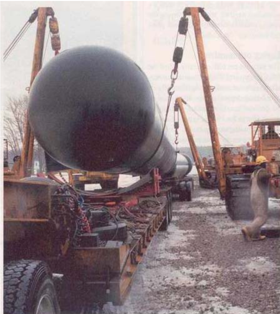
Three 62,500 gallon storage tanks lined up for unloading.
