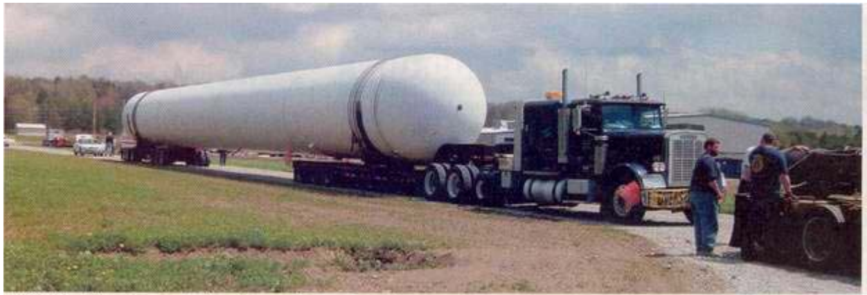
A 90,000-gallon storage tank arrives at Niagara Energy's new terminal in North Collins, N.Y. The 367,500-gallon underground storage facility was designed by Superior Energy Systems in Columbia Station, Ohio.
